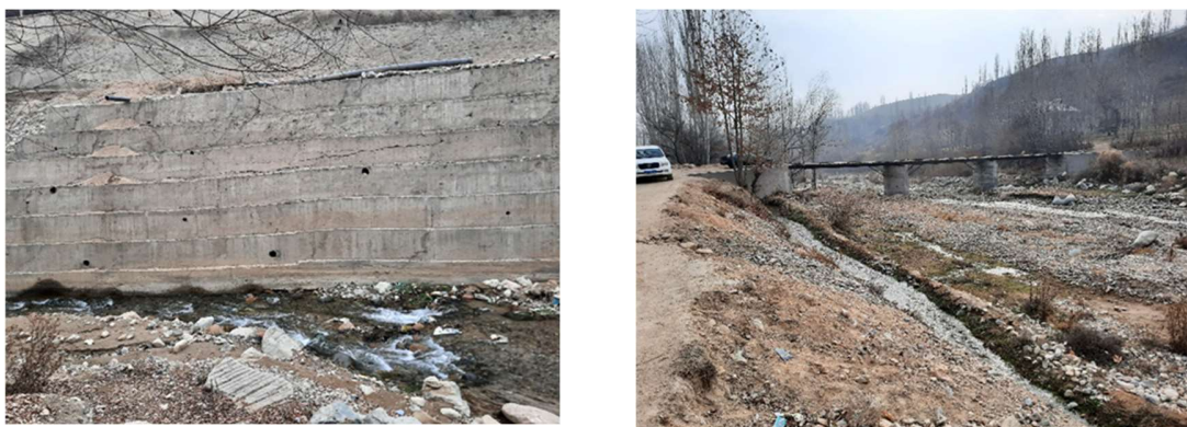
Figure 27. Isfara city, Lakon Community for Implementing Riverbank Protection Works (Tajikistan)
